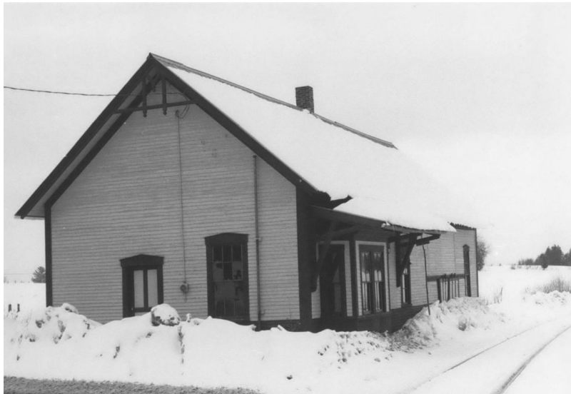
Figure 1.1 The railroad station in 1982
