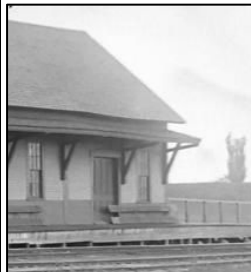
After the circa 1907 Renovation.
