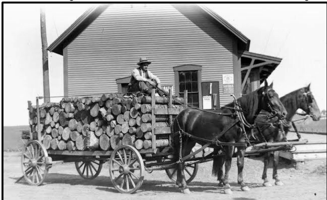
C.H. Davis with Load of Wood -1908 in Front of Danville Railroad Station.
