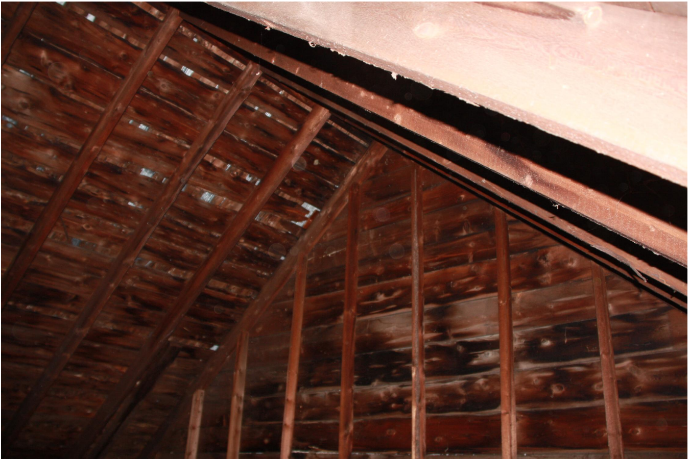
Roof looking northeast
