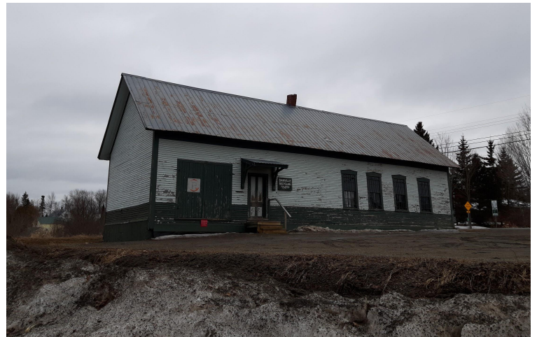
View of railroad station looking northeast
