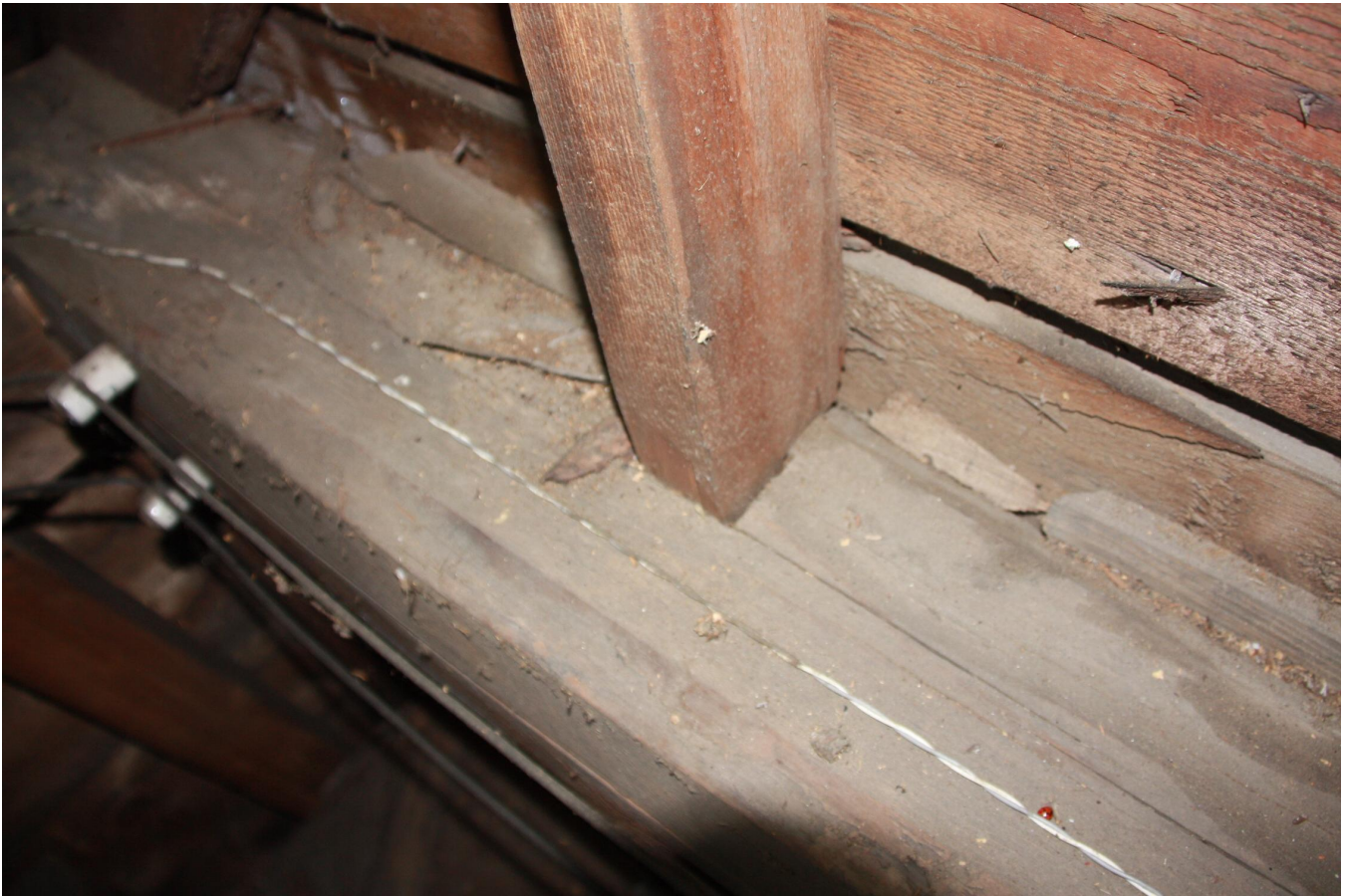
Mortise and Tenon Joint in attic looking southwest Fishburn, S. (January 2021)
