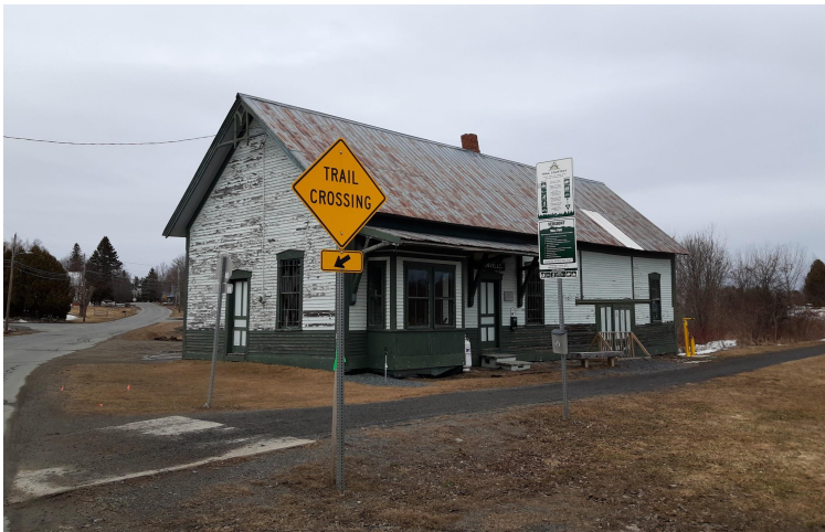
View of railroad station looking northeast
