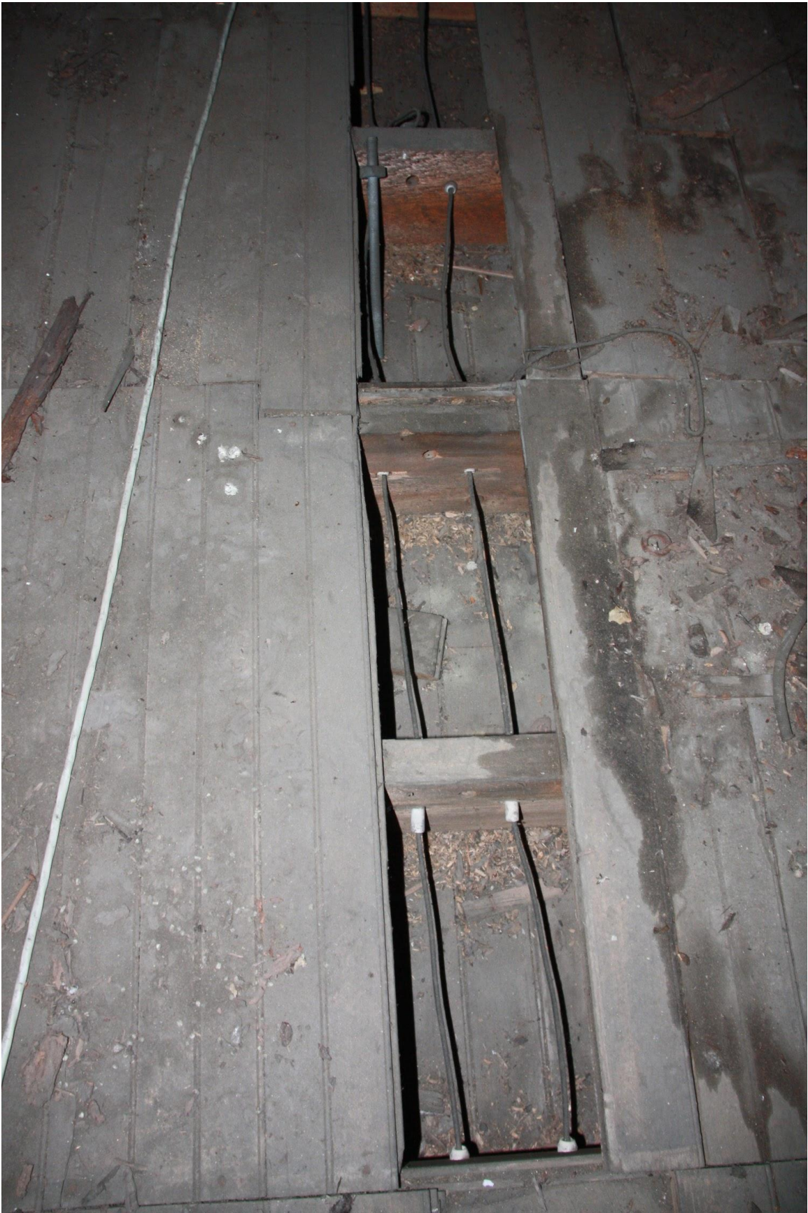
Floorboards removed in attic for electrical conduit. Fishburn, S. (January 2021)
