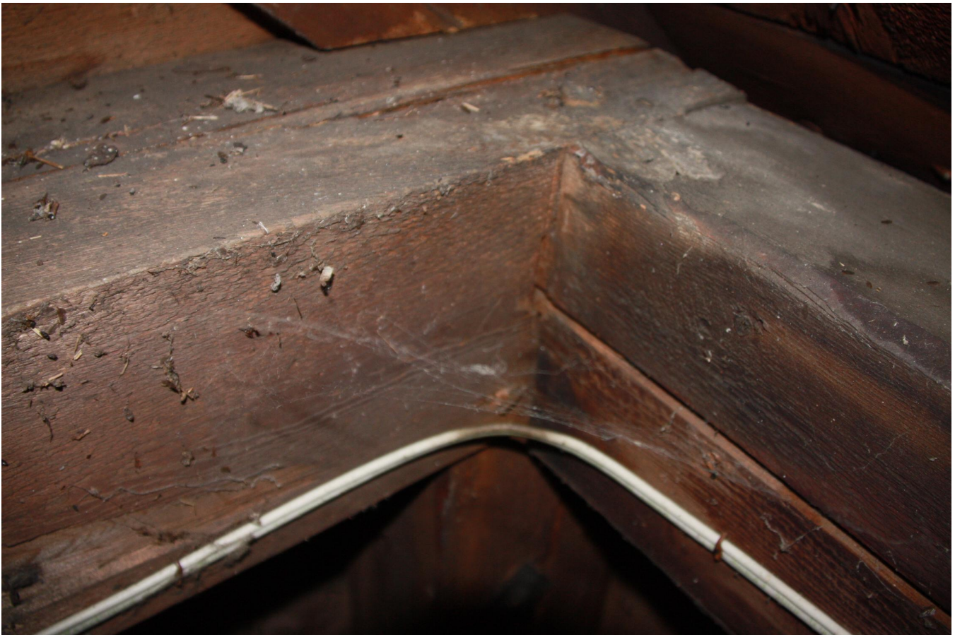
Beam Junction in attic looking southeast
