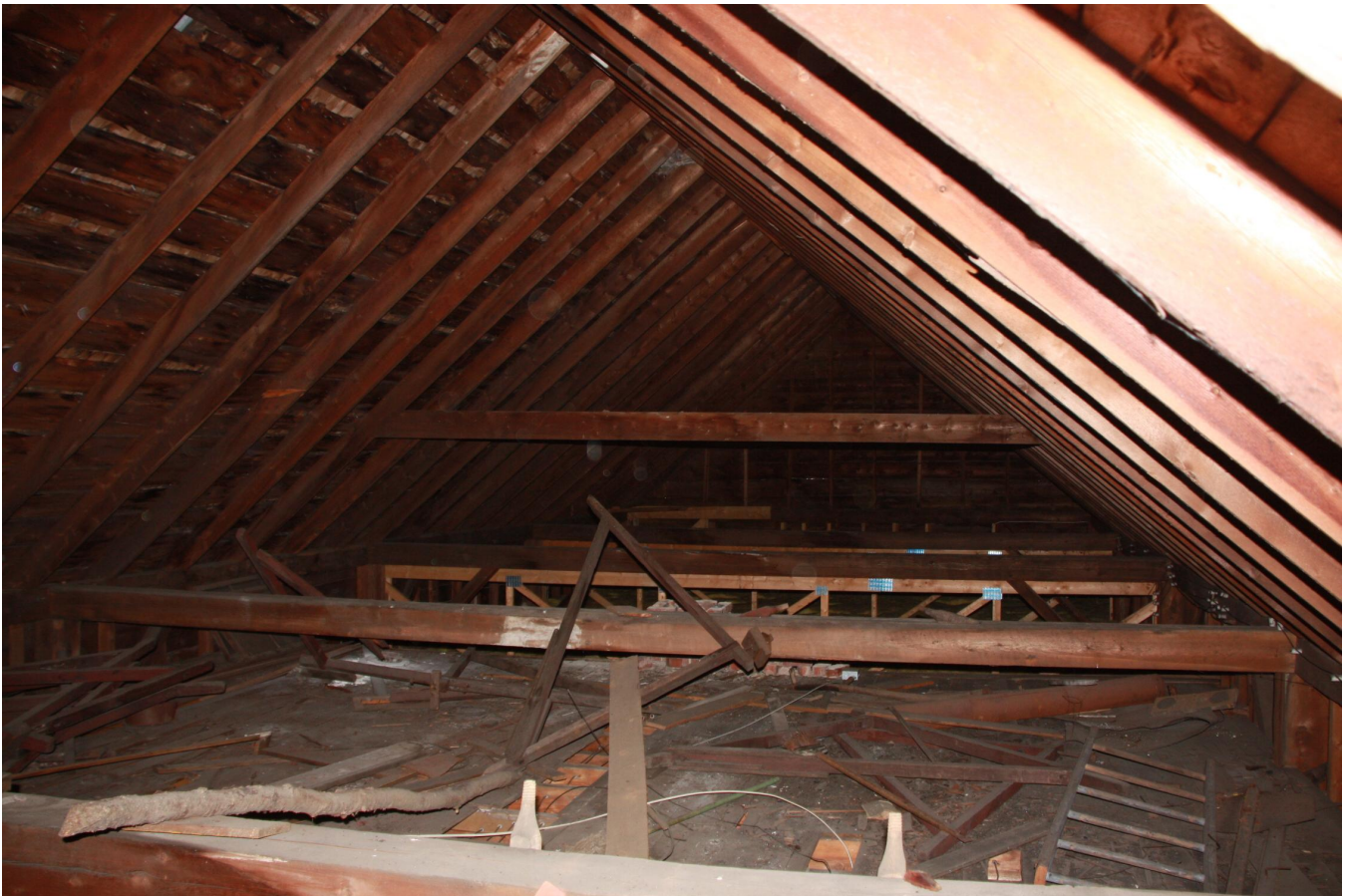
Attic looking east Fishburn, S. (January 2021)
