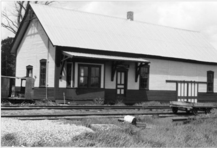
Danville Depot shortly after the 1976 renovation. -Danville Historical Society
